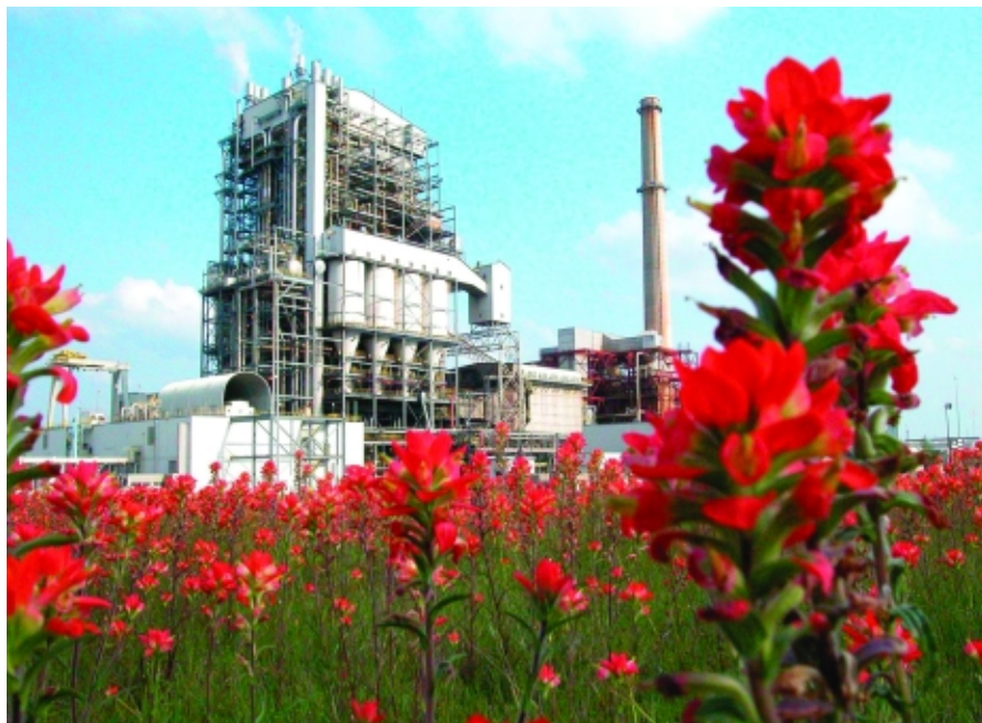
1. Gibbons Creek Station. TMPA's 480-MW Gibbons Creek Station must emit no more than 0.165 lb/mmBtu of NO x beginning in 2005. The plant began burning PRB coal in 1996. Courtesy: Burns & McDonnell
