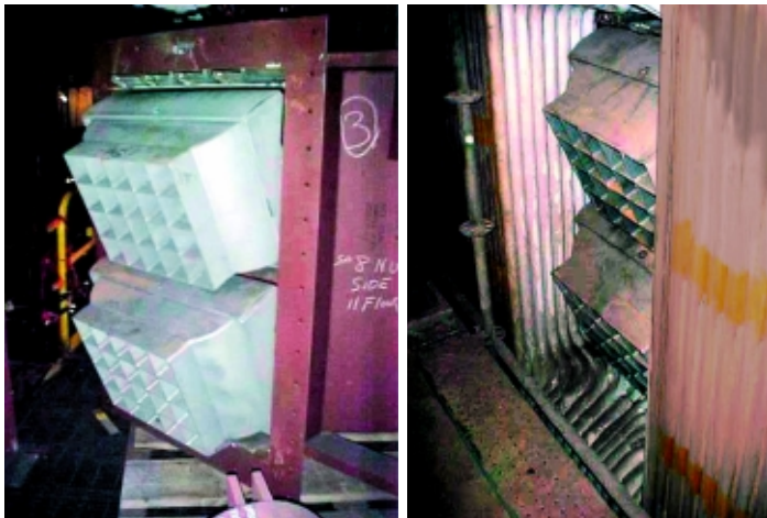
3. Close-up of a typical SOFA port assembly before (left) and after (right) installation. Adding overfire air to a tangentially fired coal-burning unit typically reduces its NO x emissions by 20% to 60%. Courtesy: Babcock & Wilcox
