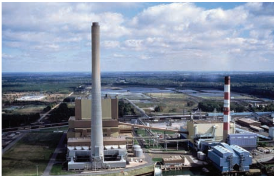
1. Upgraded for cost and environmental reasons. Consumers Energy Co.'s 265-MW J.H. Campbell Generating Station was originally designed and built by Combustion Engineering and commissioned in 1962. Unit 3 is on the left; Units 1 and 2 are on the right. Courtesy: Alstom
