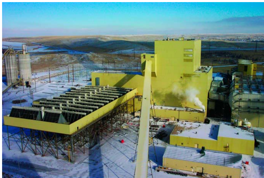
1. Now, the only dusting is of snow. A view from Wyodak's coal silo facing north-east. The large horizontal structure at left in the foreground is the plant's air-cooled condenser. Wyodak's main coal supply belts (H1 and H2) run up from the bottom through the center of the photo. Courtesy: Wyodak Power Plant
