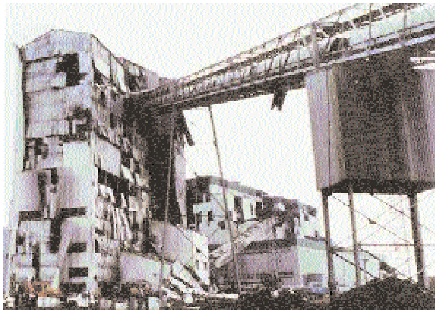
5. Secondary explosions typically cause the greatest amount of property damage, so initial response to a fire incident is critical
